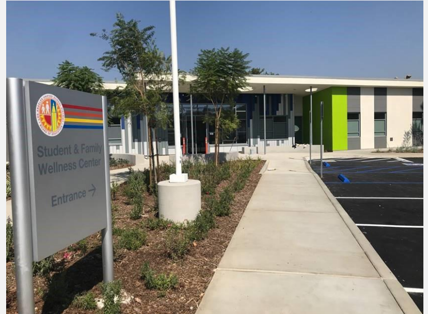
MACLAY MIDDLE SCHOOL WELLNESS CENTER WAYFINDING / PEDESTRIAN WALK TO FRONT ENTRANCE
