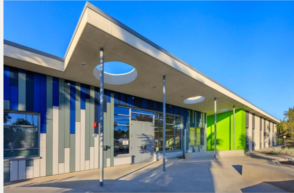
MACLAY MIDDLE SCHOOL WELLNESS CENTER WAYFINDING / PEDESTRIAN WALK TO FRONT ENTRANCE
