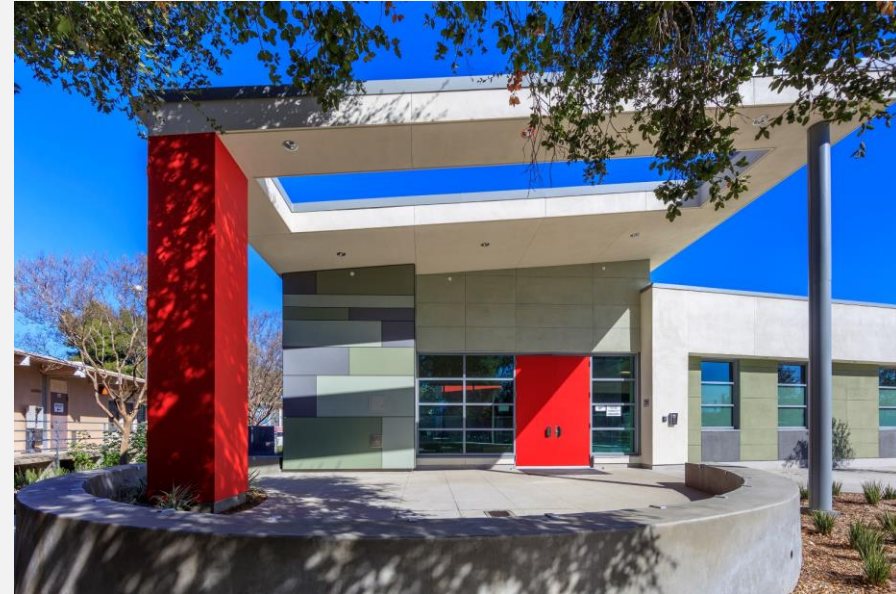
BALBOA MENTAL HEALTH CENTER FRONT ENTRANCE / OUTDOOR WAITING AREA
