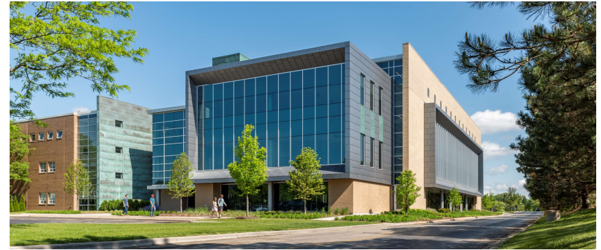
East Building Addition Phase I LEED Platinum; LAPT Platinum; Zero Energy Certified (ILFI)
